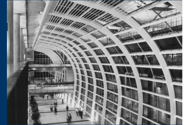
Elementy łukowe. Hong Kong Int Airport, arch. Richard Foster & Partner [6.2] (1)
